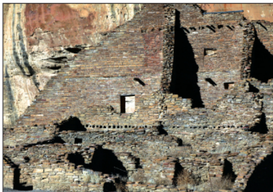
Pueblo Bonito's core-and-venter walls, and large beams of timber typifies the construction style in Chaco Canyon.
